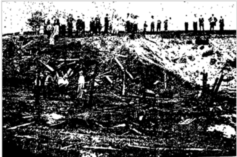
Newspaper photo of the site immediately after the explosion
